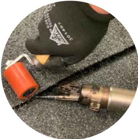
Using a heat gun, weld the laps to seal the membrane
