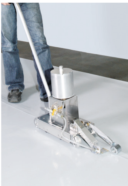
Fig. 4: welding the membrane with the alwitra solvent welding machine
