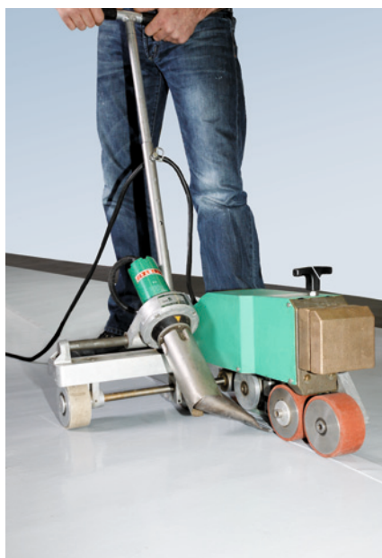
Fig. 5: welding with the hot air welding machine
