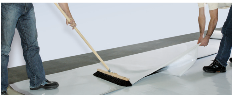
Fig. 3: pulling the protective foil to one side and pressing on, removing any blisters
