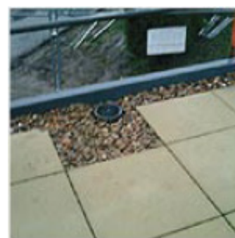
Roof patio on an office in Nottingham on asphalt system
